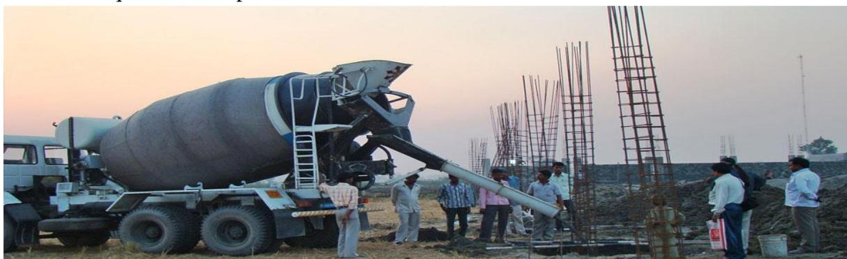
Fig3.Laying of Ready Mix Concrete
